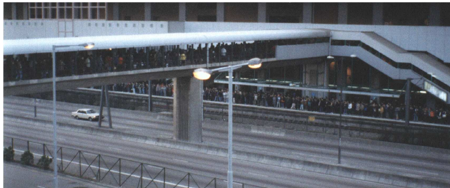
Figure 215 - View of the bridge leading from gate 3 to the platform.
