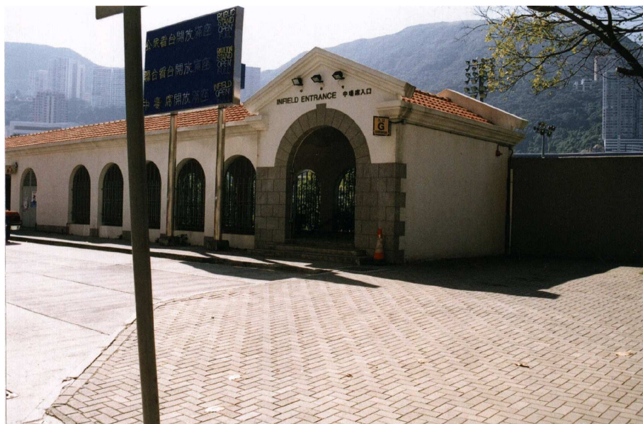
Figure 179 - The entrance to the infield tunnel. Turn left down a flight of stairs.
