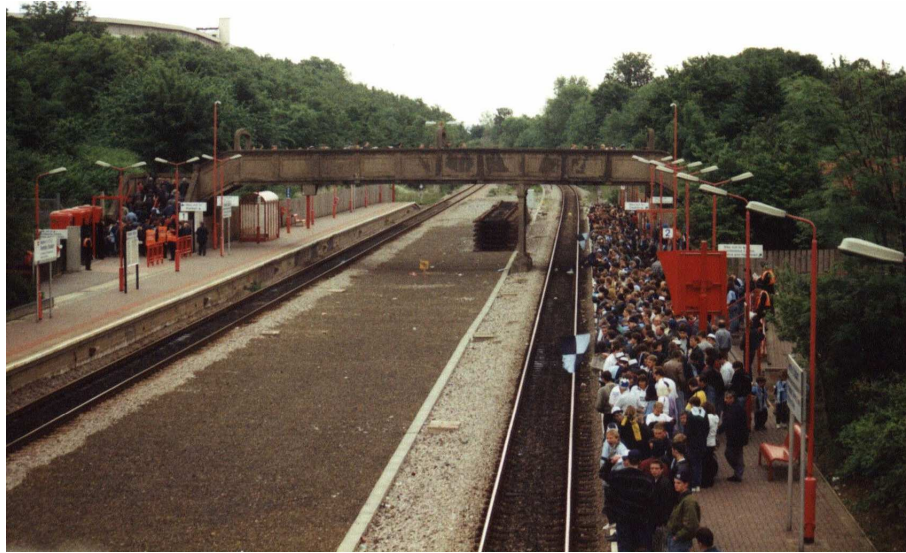
Figure 24 - Station platforms, as seen from Wembley Hill Road
