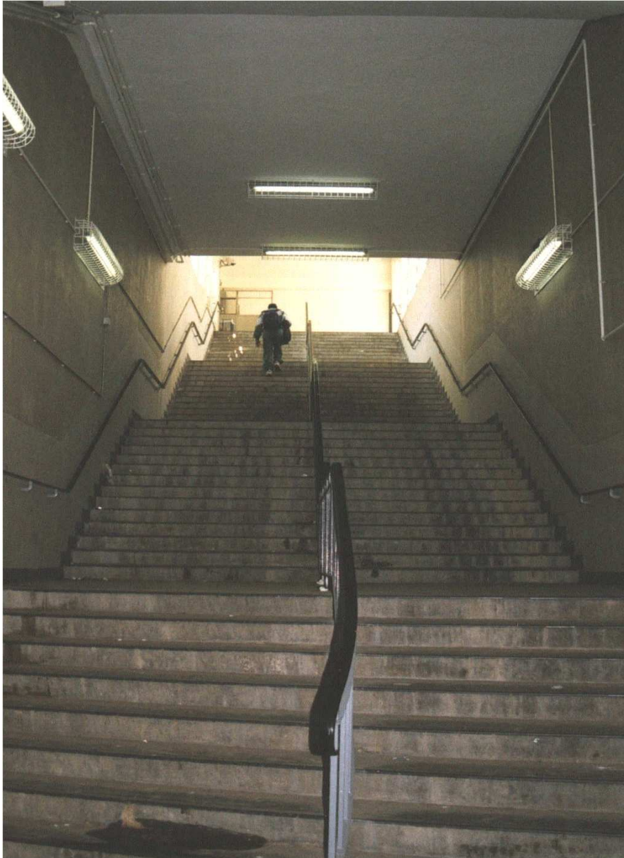
Figure 181 - Looking up the entrance stairs
