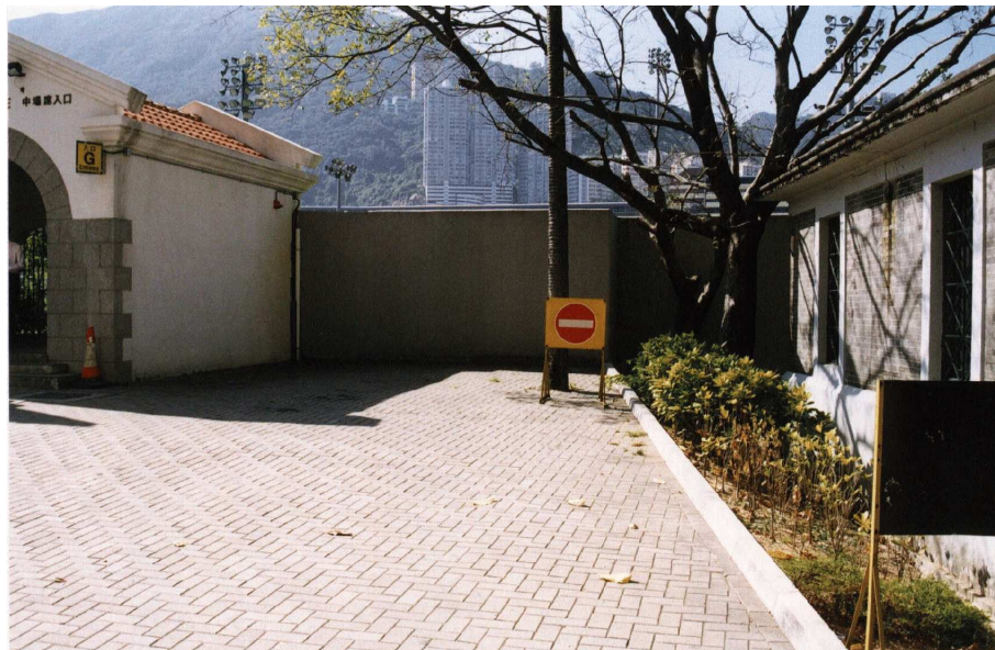
Figure 191 - The available space by the side of the infield tunnel (See Figure 182)
