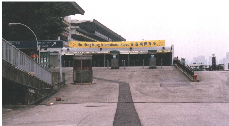
Figure 193 - The approach to gate 1 at Sha-Tin.
